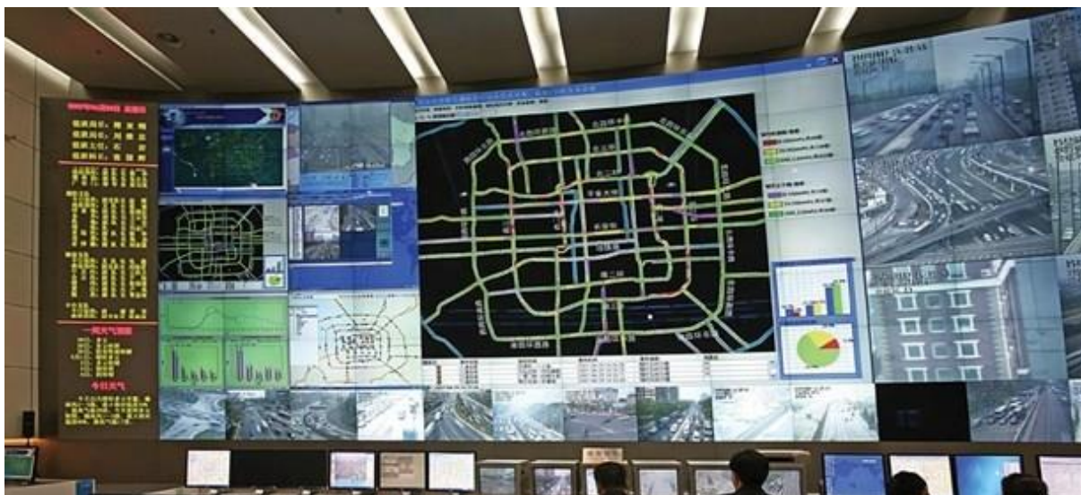
Example of control room.
